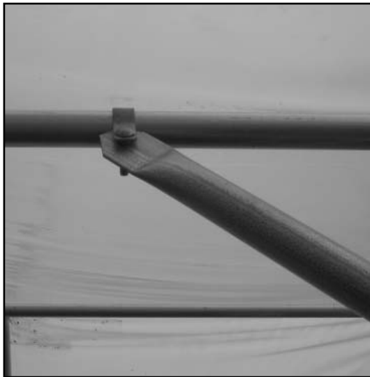
Strut Attached to Purlin
