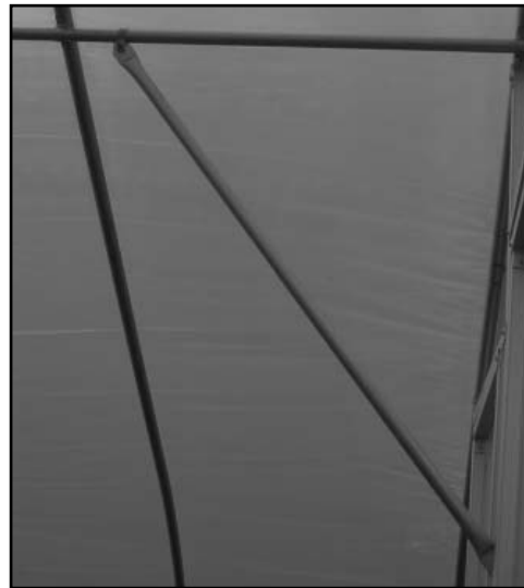
Strut from Purlin to Framing
