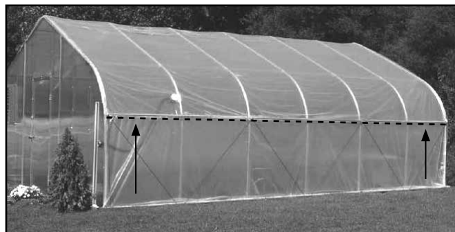
Attach main cover to Poly Latch U-Channel.
