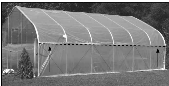
Attach main cover to Poly Latch U-Channel.
