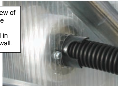
View of the intake as seen from the outside.
