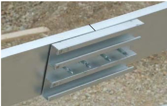
Photo shows a secured splice as seen from the back of the run of double U-channel, which is attached to the rafters.
