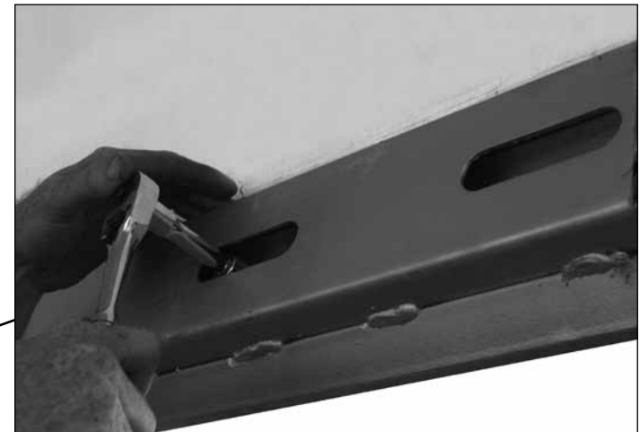
STEP 6: Tighten the coupler anchor bolts.
